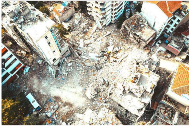
Fig. 1 collapsed building destroyed by an earthquake
